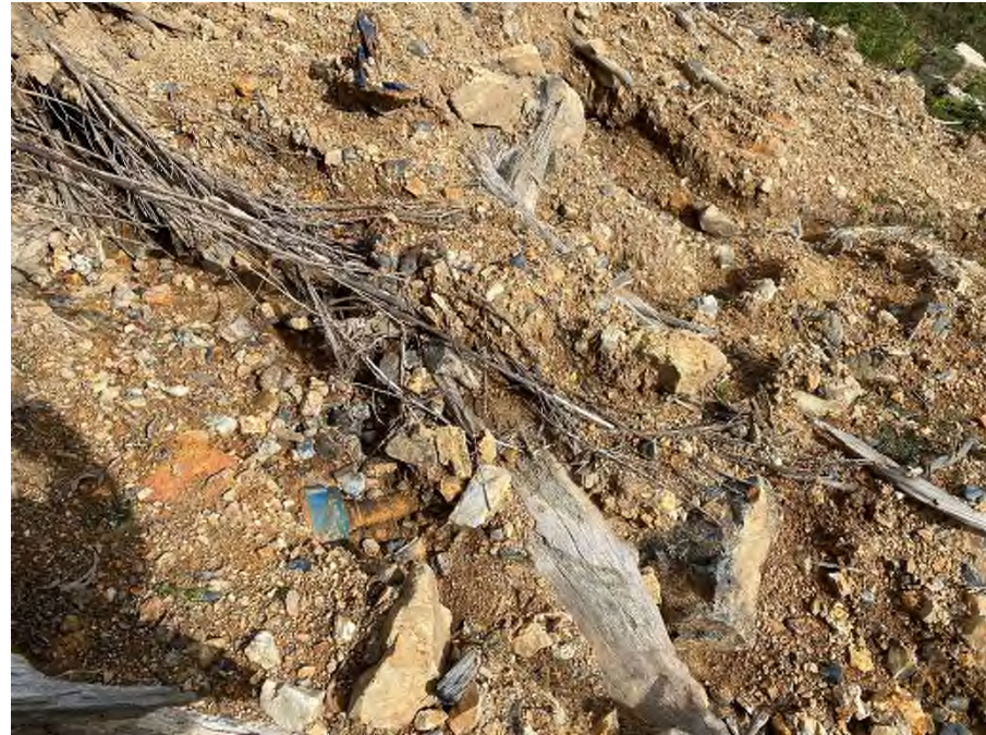
Photograph 9 , shows inert waste in fill material on northern earth bund wall. Remnants of an empty metal drum and vehicle axle are partly buried in the bund material.
