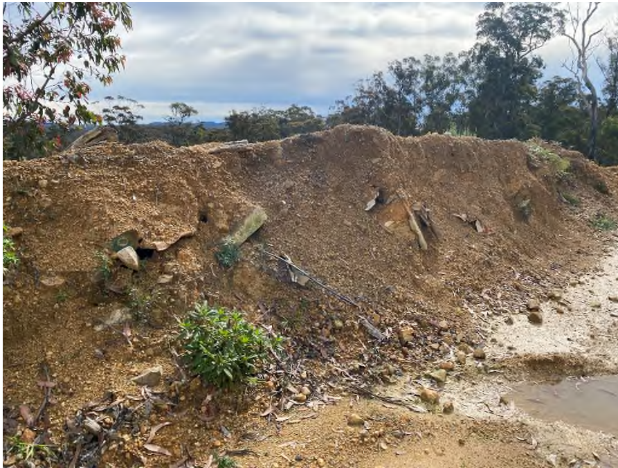
Photograph 6 , shows earth bund constructed along northern extent of the quarry pit. Visible inert waste can be seen within this bund including; concrete, and metal items.
