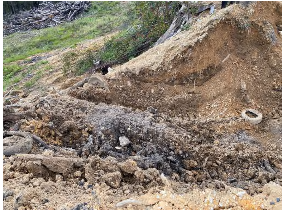
Photograph 7 , shows area in central portion of the northern earth bund which has been previously excavated. Several previously buried tyres can be seen in the photograph.
